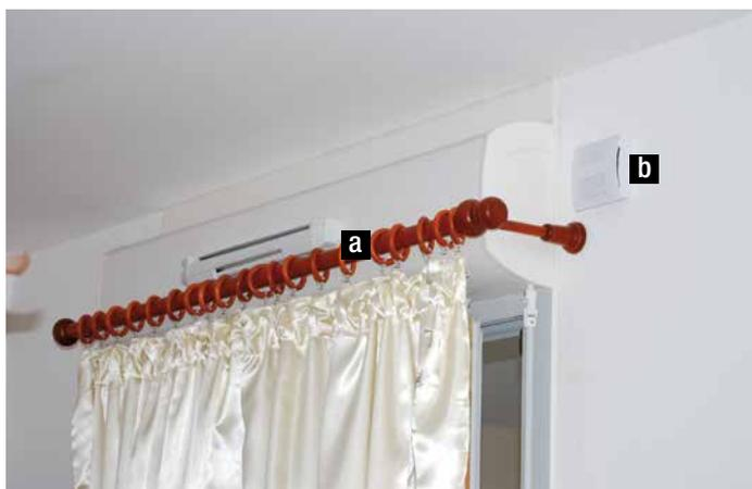
Aereco humidity controlled air inlet on a rolling shutter casing **a**. Humidity, temperature and CO<sub>2</sub> sensor **b**.
