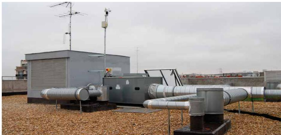
On the roof, centralised fan and weather station for wind and external conditions (temperature, humidity and CO<sub>2</sub>).
